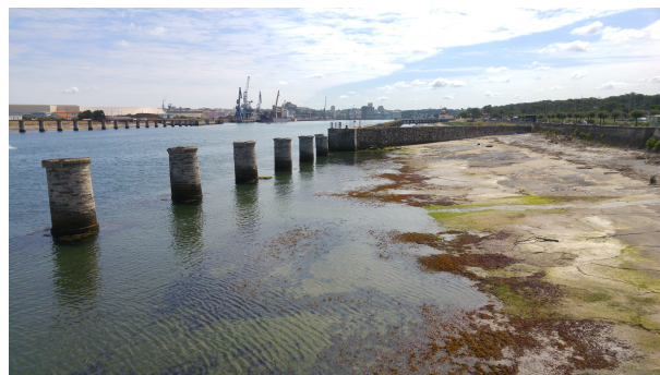
Figure 2.8 – Expansion area (left bank) (2016).
