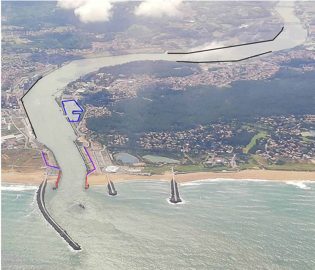
Figure 2.7 – Aerial photo of the Adour river mouth: (at the forefront, from left to right) north, middle and south breakwaters, (red lines) convergent and (purple lines) expansion areas. (black lines) River seaport terminals: (left) Tarnos, (lower right) Blancpignon and (upper right) Saint Bernard. (blue lines) Marina. Photo by Sophie Defontaine (2019), reproduced with permission.
