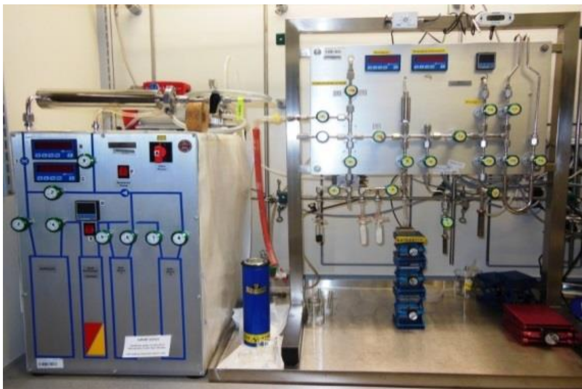
Figure 4: The tritium manifold
