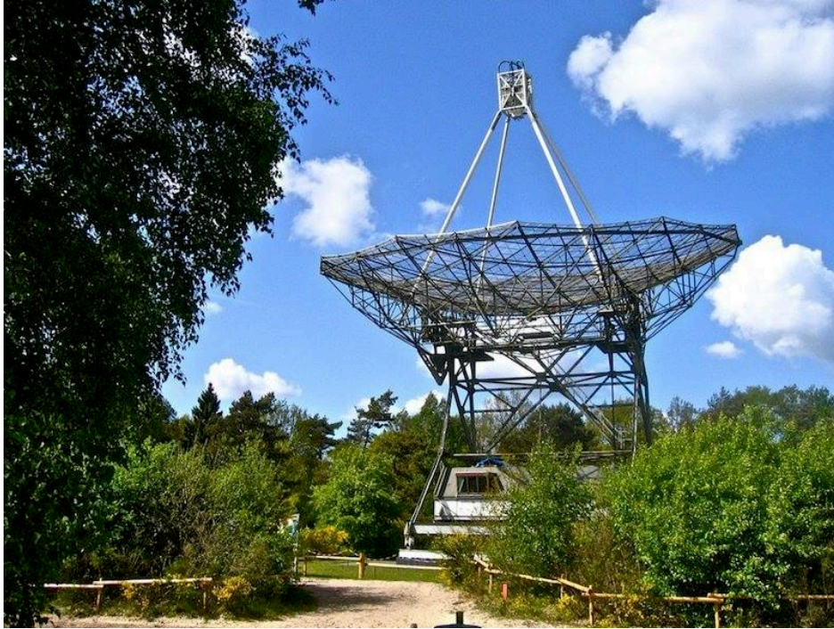
Figure 9.5: The 25 m antenna of the station PI9CAM, in Dwingeloo, Netherlands.
