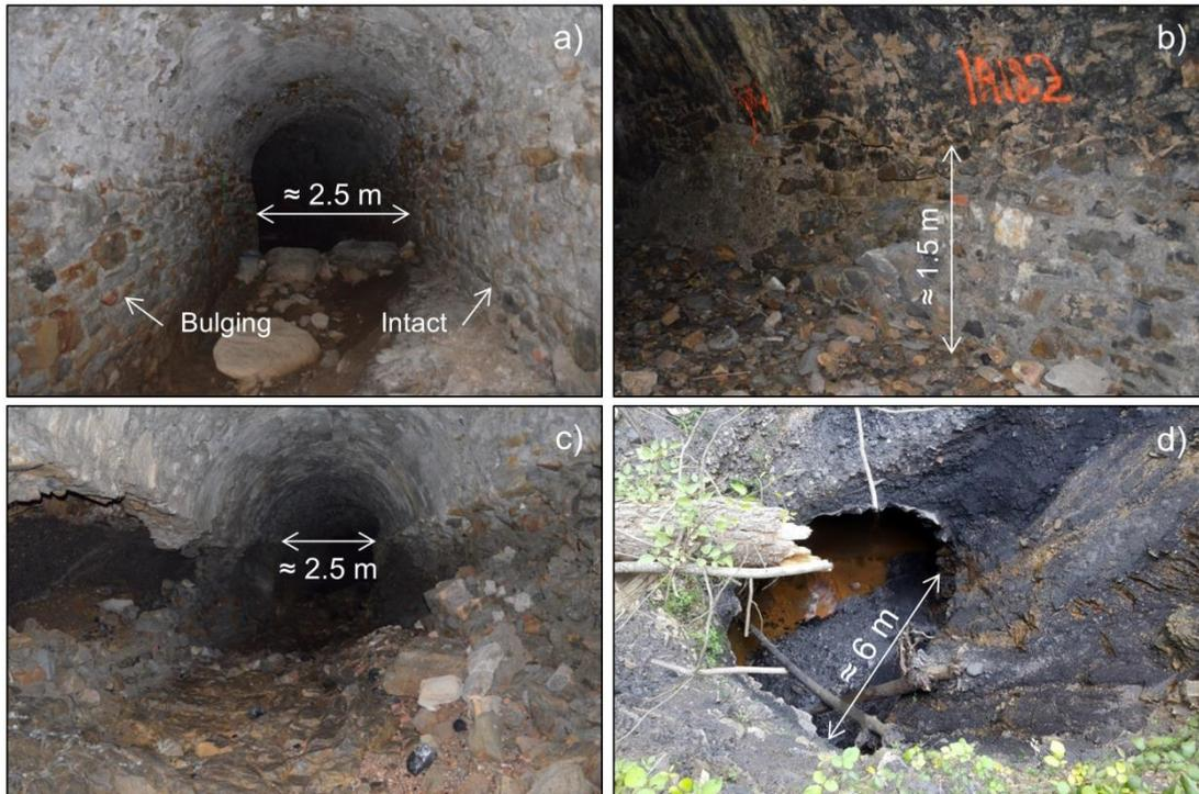
Fig. 5: Photographs taken during summer 2017: a) intact and bulging sidewalls inside *La Vieille Valette* CS tunnel (Robiac-Rochessadoules, France) ; b) cracking sidewall inside *La Valette* CS tunnel (Robiac-Rochessadoules, France) ; c) collapsed sidewalls in *La Vieille Valette* CS tunnel (Robiac-Rochessadoules, France); d) collapse of the sidewall, the vault and the surrounding soil above *Chamclauson-1* CS tunnel (La Grand-Combe, France).
