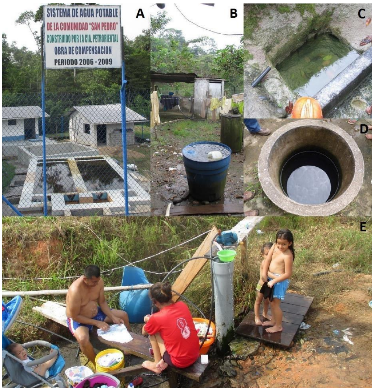
Figure VIII. Domestic water sources in Ecuador: A. Treated piped water network. B. Rainfall water collected in plastic tank. C. Spring water. D. Artesian private well. E. Deep public well. (Photo Credits : MONOIL®, 2016).
