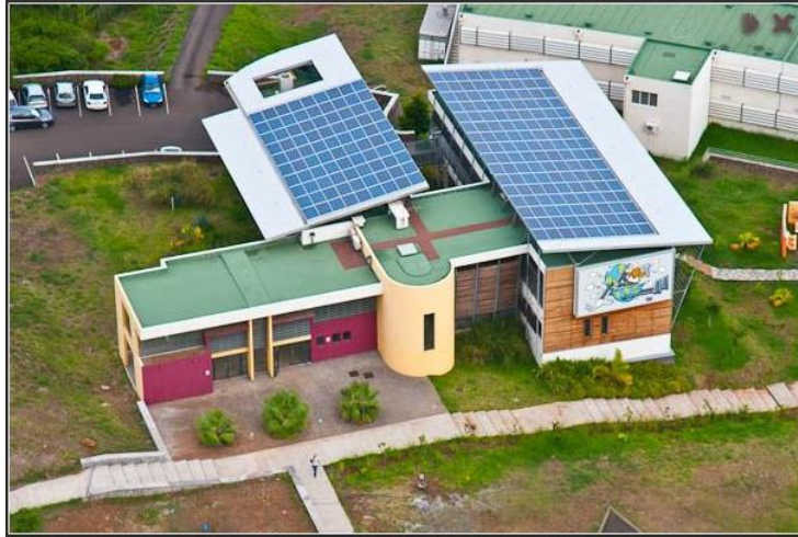
Figure A- 7. BIPV roof on ENERPOS. 365 m 2 of PV panels to balance the low consumption of the building. Picture credits: Jerome Balleydier.
