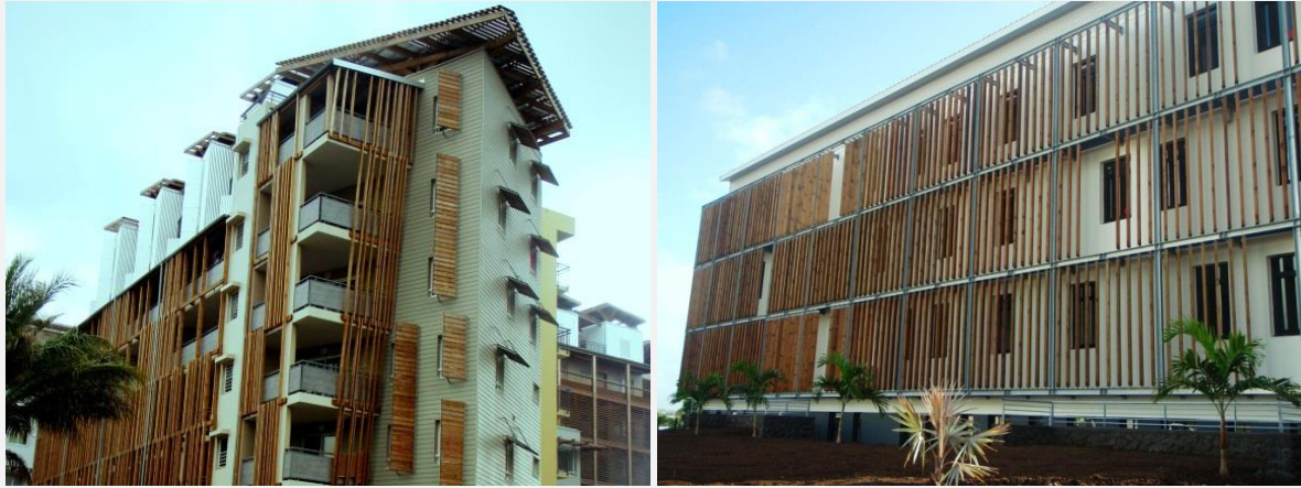
Figure 1-19. Examples of fixed solar shading. Left: Residence of Flores-Malaca, Le Port, Reunion Island. Architects: Antoine Perrau / Michel Reynault. Right: Head office of CIREST, Saint-Benoit, Reunion Island. Architects: Sylvain Guy / Guillaume Hazet.
