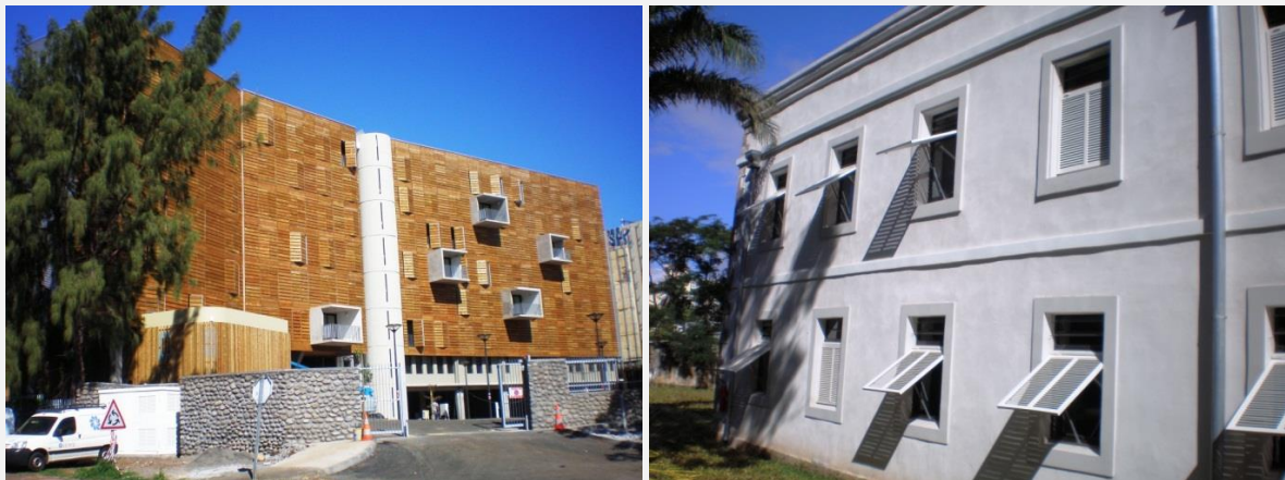
Figure 1-20. Examples of mobile solar shading. Left: University housing and offices of CROUS, Saint-Denis, Reunion Island. Architects: T & T architecture. Right: Head office of DIREN, Saint-Denis, Reunion Island. Architect: Olivier Brabant.
