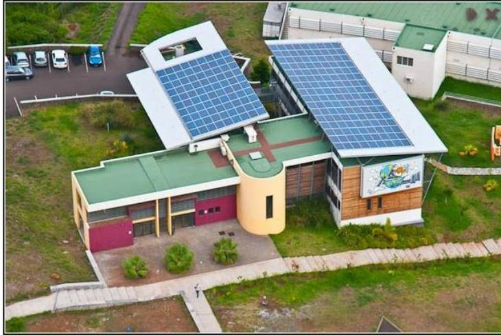
Figure A- 7. BIPV roof on ENERPOS. 365 m<sup>2</sup> of PV panels to balance the low consumption of the building.
