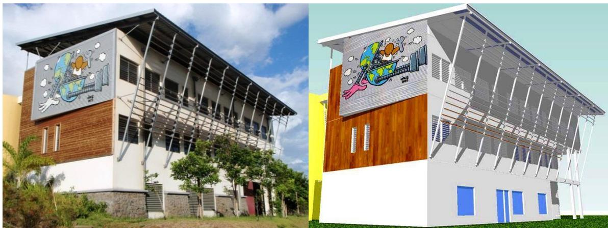
Figure 4-1. Comparison between a picture of the ENERPOS building (November 26<sup>th</sup> at 5 p.m.) and the SketchUp Model with projected shadows of shading at the same time.
