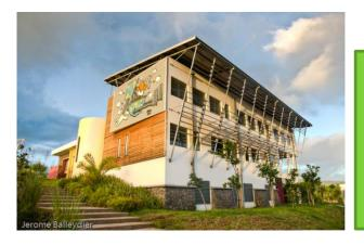
**Technical data:** Net Floor Area: 739 m<sup>2</sup> Gross Floor Area: 1,425 m<sup>2</sup> Conditioned Area: 246 m<sup>2</sup> (33% of the NFA) 2 buildings – 2 floors PV:  $365m^2 - 50$  kWp Construction completion: July 2008 Cost:  $3.200 \notin m^2_{NEA} = 1.660 \notin m^2_{CEA}$
