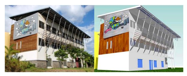
Figure 4-1. Comparison between a picture of the ENERPOS building (November 26<sup>th</sup> at 5 p.m.) and the SketchUp Model with projected shadows of shading at the same time.
