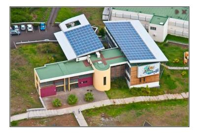
Figure A- 7. BIPV roof on ENERPOS. 365 m<sup>2</sup> of PV panels to balance the low consumption of the building. Picture credits: Jerome Balleydier.
