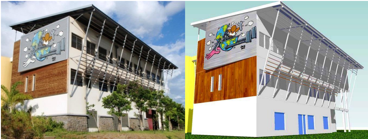
Figure 4-1. Comparison between a picture of the ENERPOS building (November 26 th at 5 p.m.) and the SketchUp Model with projected shadows of shading at the same time.
