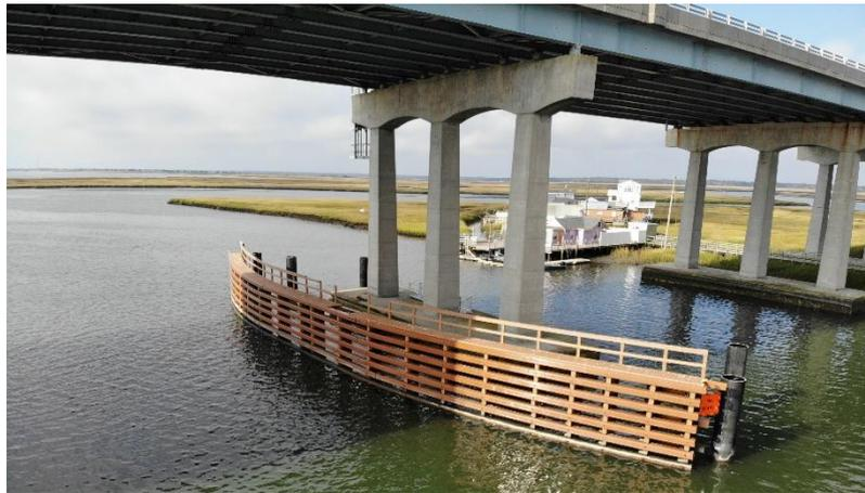
**Figure II.6:** Fender system for bridge pier protection (source: <https://www.compositeadvantage.com>).
