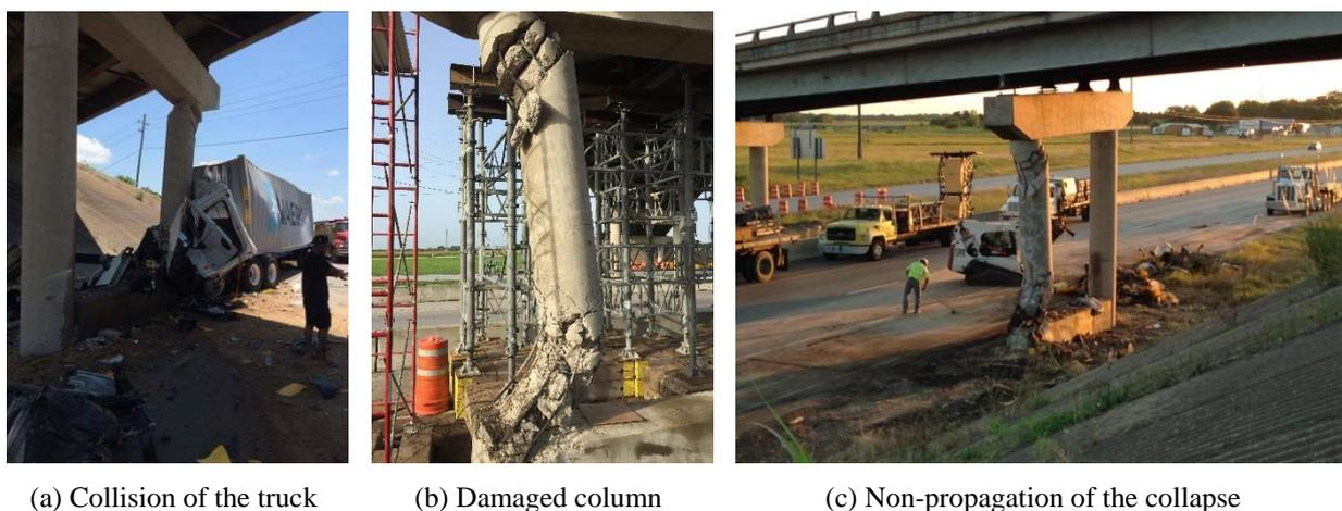
**Figure I.8:** I-10 bridge collision (source: <https://www.aggregatetechnologies.com/>).
