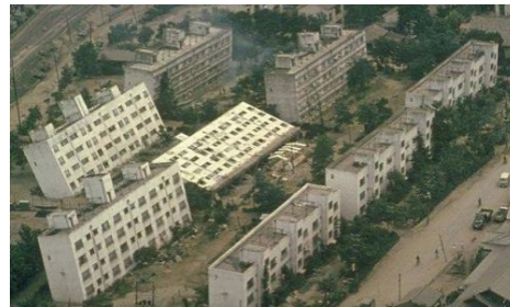
(b) Liquefaction at Niigata
