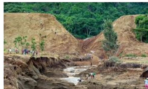
(b) Broken banks of the Patel dam, Kenya
