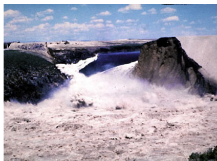
(c) Teton dam failure
