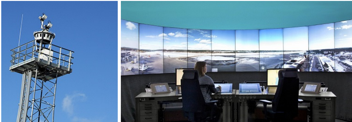
(a) RCT equipment installed at Örnköldsvik airport. (b) RCT installation at Sundsvall to remotely control Örnköldsvik and Härnös airports.
