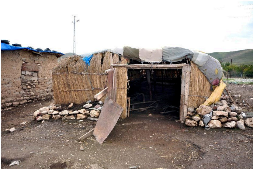
Figure 5.124: Architectural change of Wattle Structures to Stone-Walled Wattle Structures in Memika Kom
