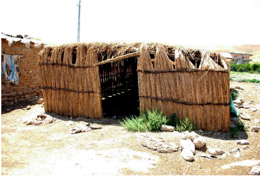
Figure 5.123: Wattle Structures in Memika Kom
