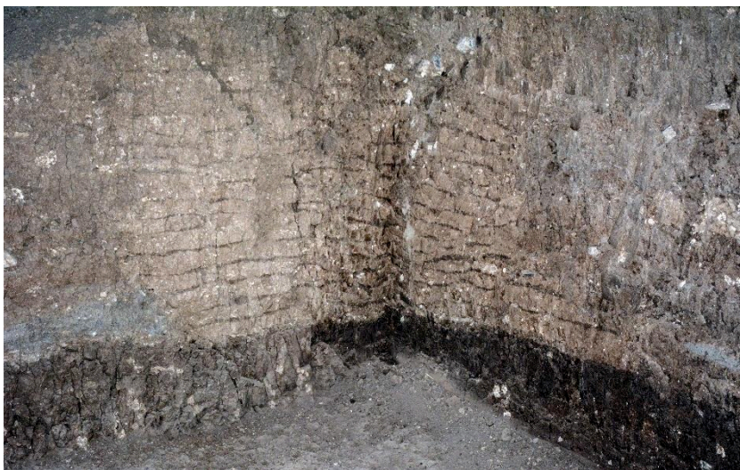
Figure 4.104: Cross-section of massive piled earth (Structure N6B4)
