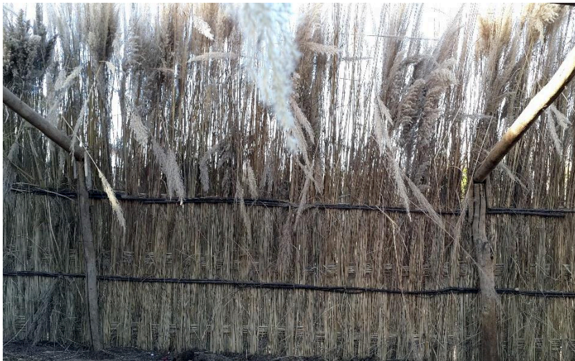
Figure 5.42: Some wooden poles in a Wattle Structure, near Kumgeçit village
