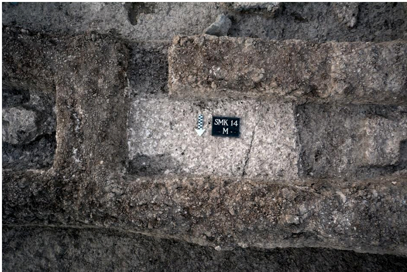
Figure 4.124: Massive piled earth walls and lime traces on the cell base of Structure N6B10
