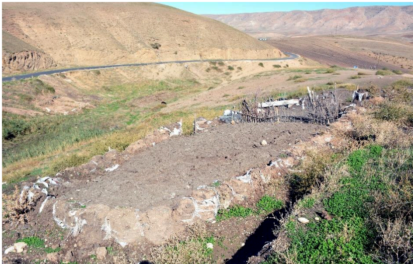
Figure 5.128: Example of Earth Wall (Piled Earth) in Mezrik Kom
