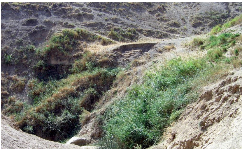
Figure 3.40: Current landslide traces, on the northeastern slope of Sumaki Höyük
