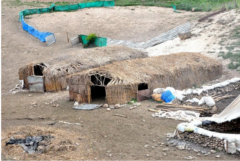
Figure 5.102: Front view of some Wattle Structures in the Area 2 from Bazivan Kom
