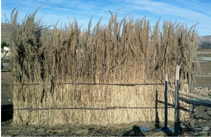
Figure 5.41: Architectural construction process of a Wattle Structure, near Kumgeçit village
