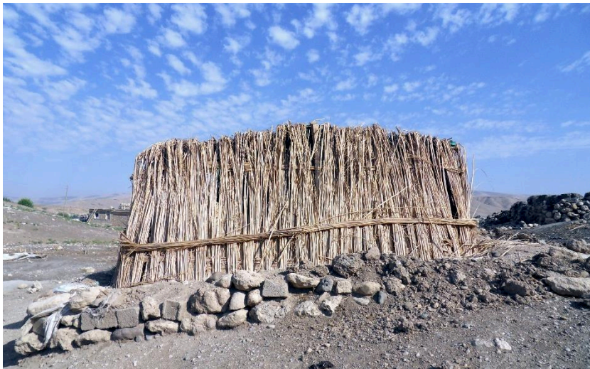
Figure 5.49: Stone-Walled Wattle Structure in Bazivan Kom, south of Kumgeçit village
