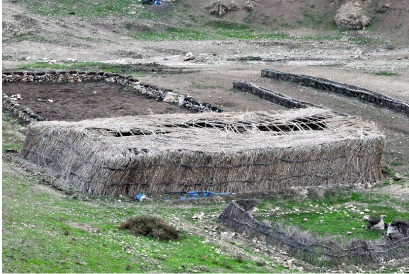
Figure 5.105: General view of some Wattle Structures in the Area 1 from Bazivan Kom
