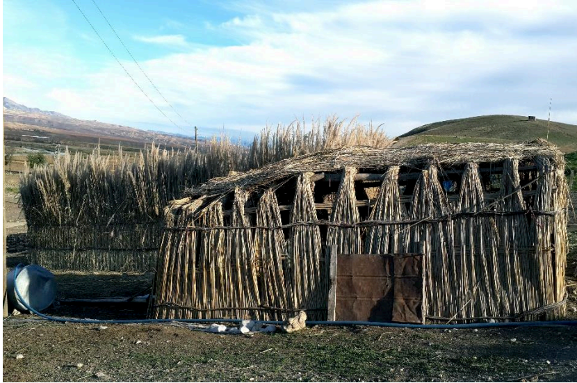
Figure 5.38: External view of the Wattle Structures and its architectural construction process, near Kumgeçit
