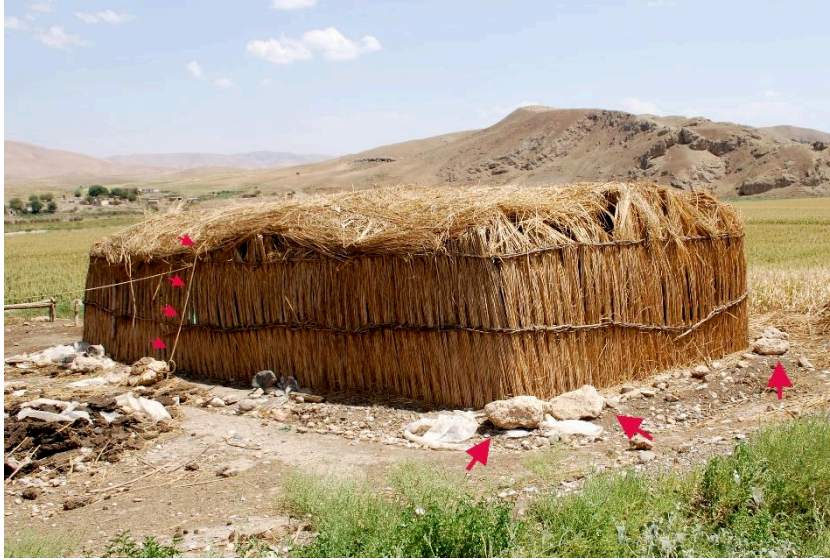
Figure 5.32: External view of Memika Saz Evi and its tensioning system, near Gedikli village
