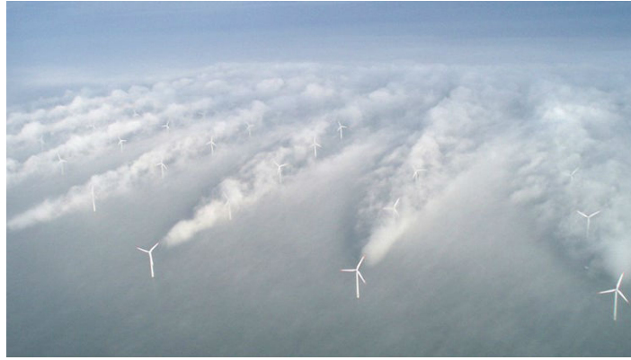
Figure 2.12 — Example of wake effect [57].
