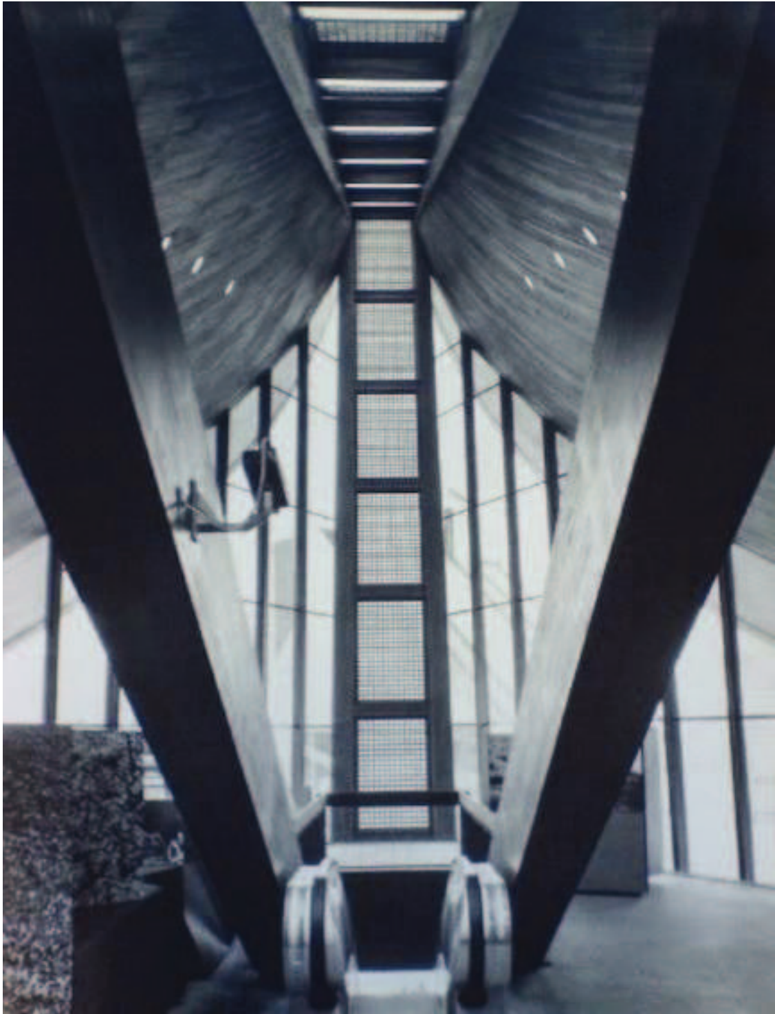
Illustration n° 264 : Pavillon des Philippines, 1970. Nicholas Polites, The Architecture of Leandro V. Locsin . New York: Weatherhill, 1977.
