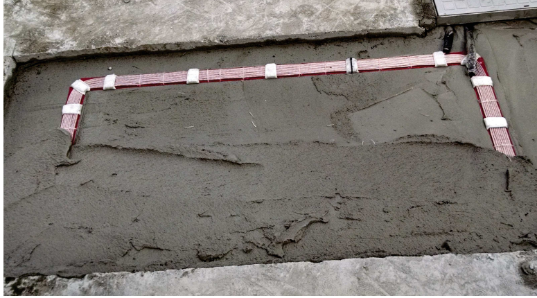
Figure 5.11: Road-embedment of the 9-turns WPT in dry concrete.
