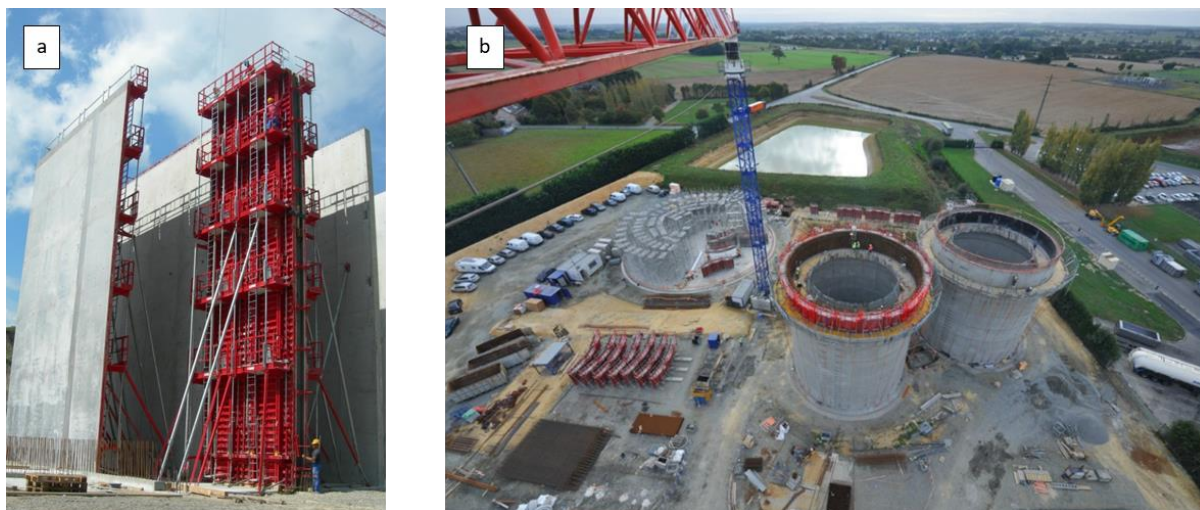
Figure 3 : a) Coffrages plans traditionnels : Coffrages H12, FRUTIGER (CH), Bern, 2012, ©MCA, © Hussor.com, b) coffrages cintrables : Coffrages C12-10, GTM Ouest, Valdis, 2011, © Willy Berre, © Hussor.com
