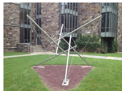
Figure 3.8: Tensegrity structure with cables under extension and rods under compression. A Snelson-Fuller sculpture in the graduate college courtyard at Princeton.
