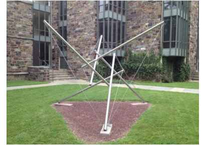
Figure 3.8: Tensegrity structure with cables under extension and rods under compression. A Snelson-Fuller sculpture in the graduate college courtyard at Princeton.
