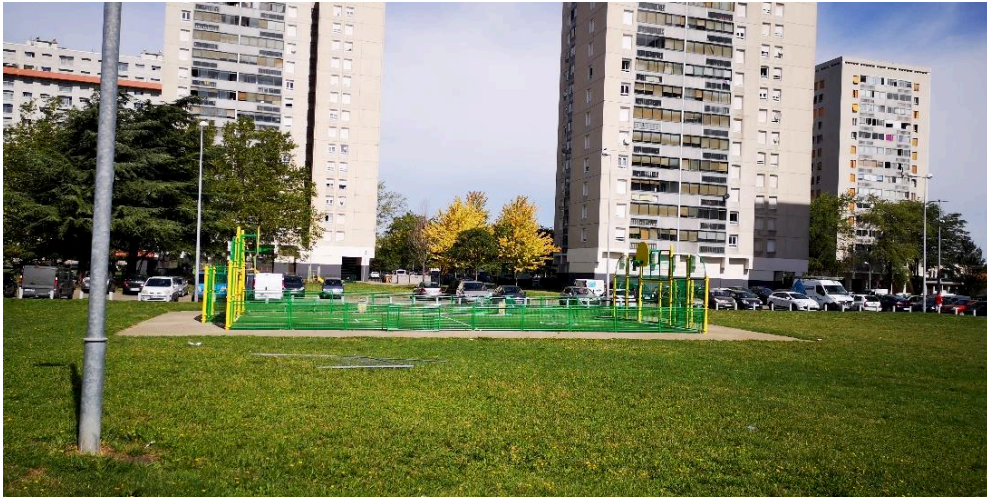
Photo 15: One of basketball courts
