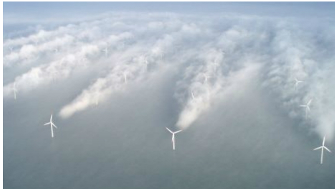
Figure 1.6: Wind farms wake effects: clouds appearing in the wake of WTs at the Horns Rev wind farm (Denmark). Picture taken by Christian Steiness, 12 February 2008.
