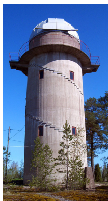
Fig. 3.15. — Tuorla Observa- tory in Finland.
