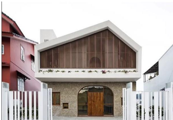
Photo 2.51: La façade moderne Source : Truong An Architecture , 2019
