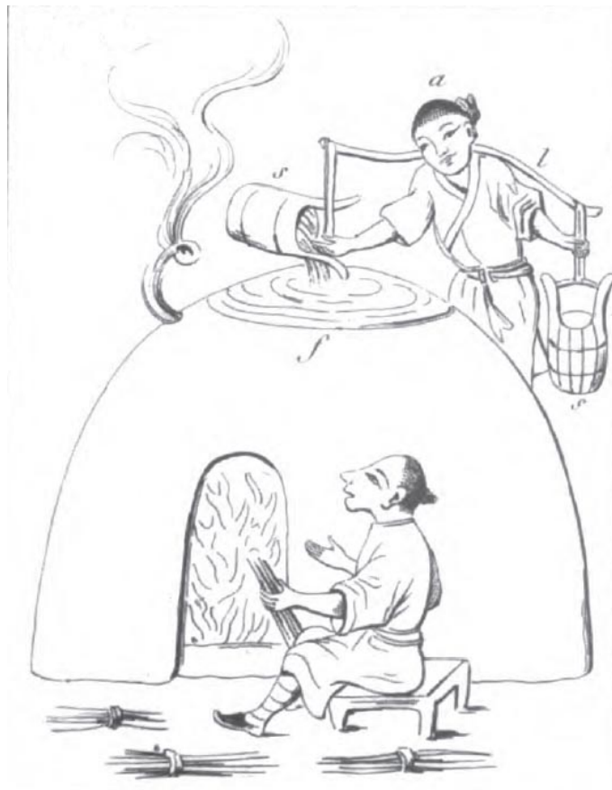
Figure 2.55: Chinese kiln for firing tile and brick with glazes, the glaze layer was produced by treatment during firing
