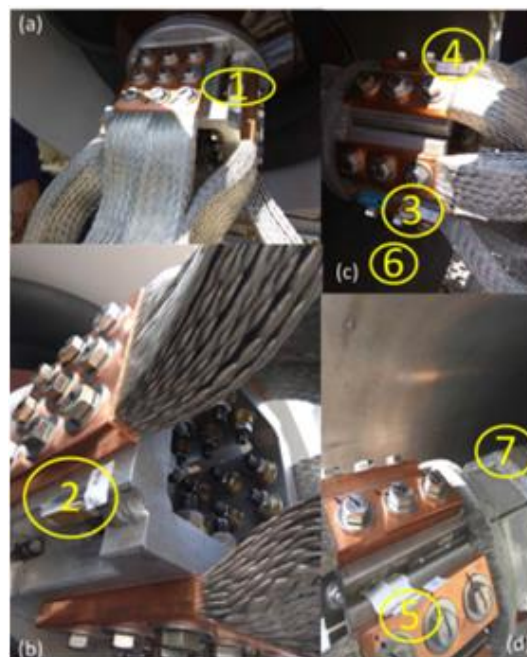
Figure 7.17: Installation positions of the RFID sensor tags in each transformer connection (seven positions overall)
