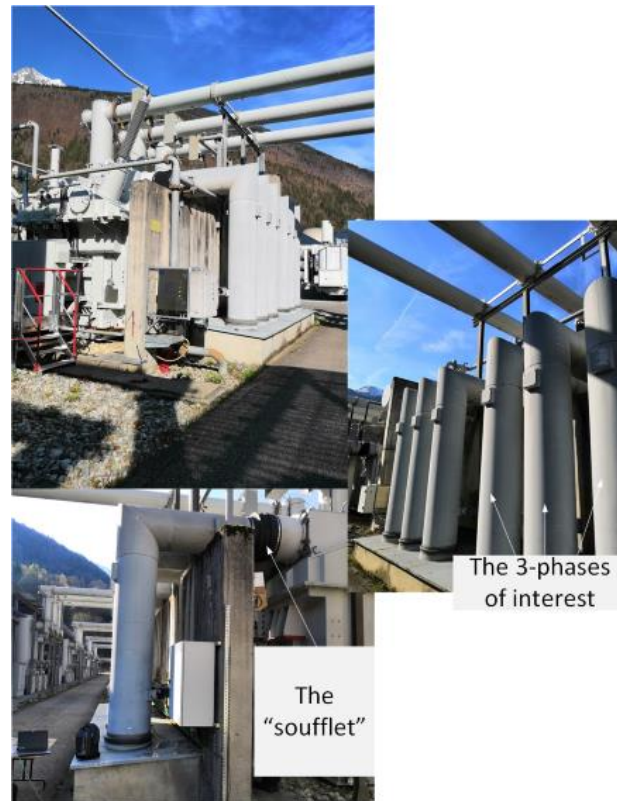
Figure 7.14: Transformers in hydroelectric power-plant of Grand'Maison
