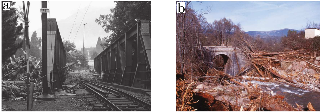
Figure I.1: Wood accumulations near a bridge (a) in Sarnen, Switzerland, during 2005 flood (Schmocker & Hager, 2011) and (b) in Venero Claro, Spain during 1997 flood (Ruiz-Villanueva et al. , 2013) both caused significant economic losses.
