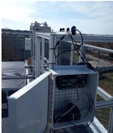
Figure 141 Installation de la centrale d'acquisition
