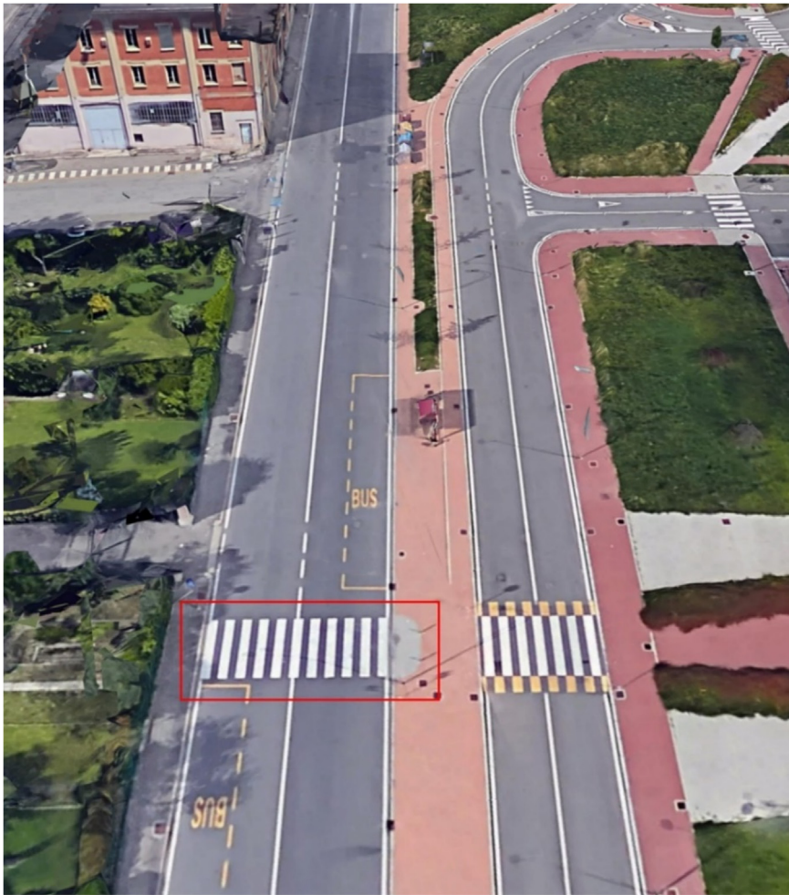
Fig. 5. Aerial view of the experimental pedestrian crossing considered in the study.
