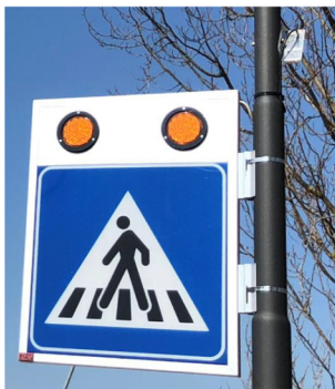
Fig. 3. Components of the integrated lighting-warning system: LED strips on both curbsides of the zebra crossing; backlit pedestrian crossing sign with flashing orange lights; dedicated lighting that enhanced the light power when the sensor detected a pedestrian. (For interpretation of the references to color in this figure legend, the reader is referred to the web version of this article.)
