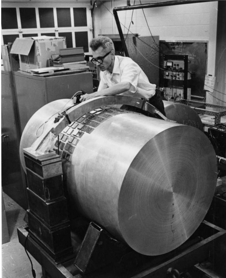
Figure 2.1 – Joseph Weber with an aluminum bar instrumented with piezoelectric crystals to read out the vibrations.
