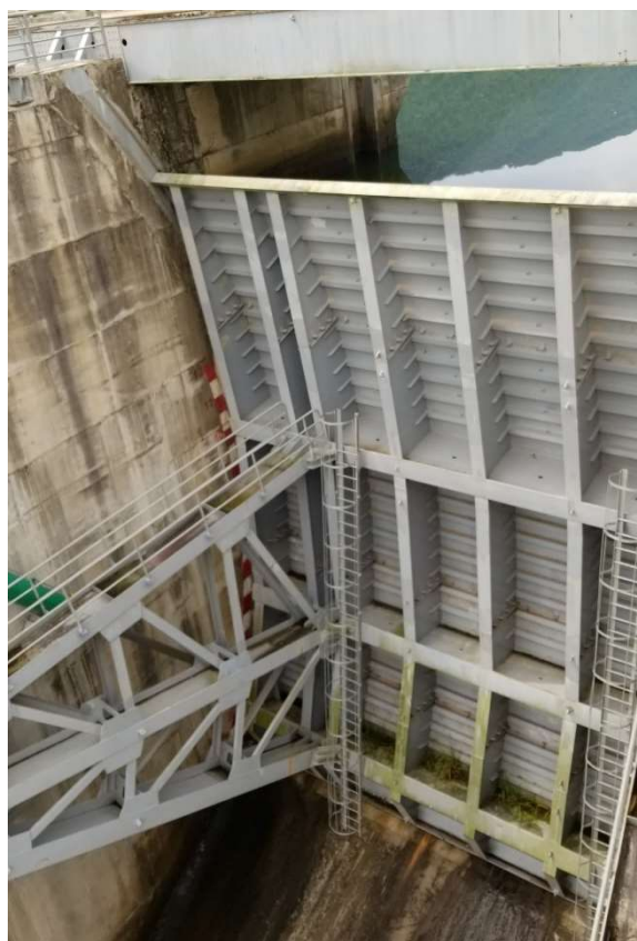
Figure 2.8. A radial gate of A Vuong spillway.
