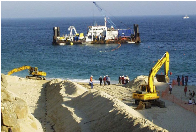
Figure 4: . Installation works of the 2000 FLAG Atlantic 1 in the intertidal area, Brittany, France (courtesy: www.ldravocean.fr ).
