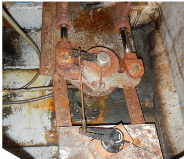
Figure 2.10.: Steven Paul's steering system and rudder angle sensor
