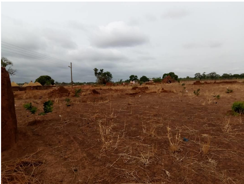
Figure 22: A cluster of houses belonging to one side of the conflict destroyed and abandoned
