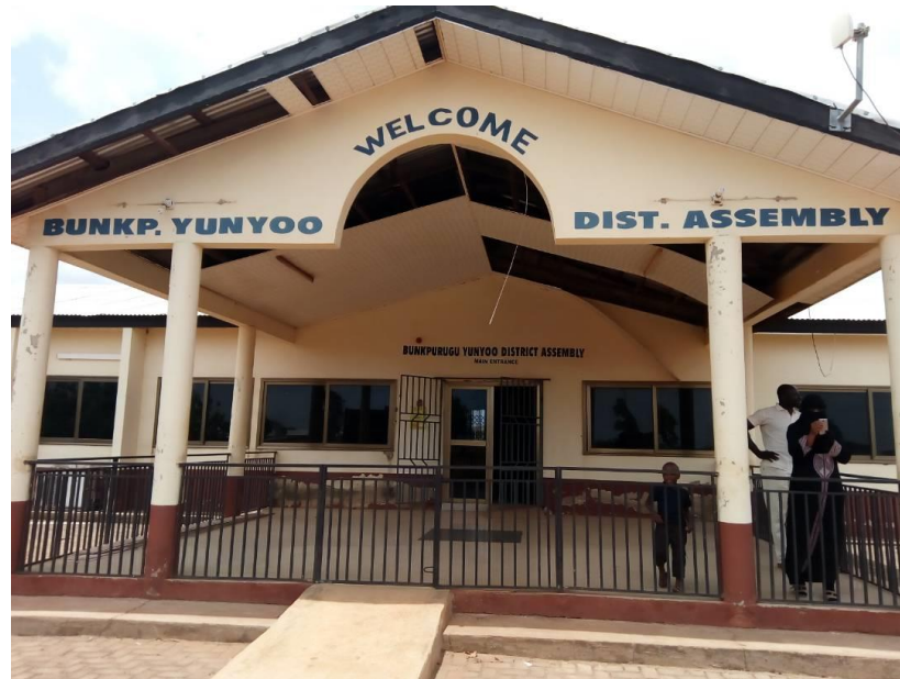
Figure 17: Bunkpurugu-Yunyuo District Assembly Building, located in Bunkpurugu (source: taken by researcher, April, 2018)
