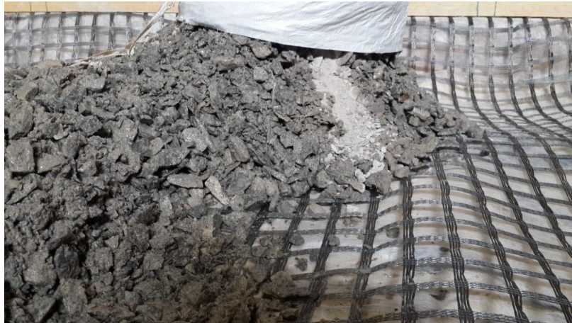
Figure 2.3-16: Installation of the GSY 1 and aggregates.
