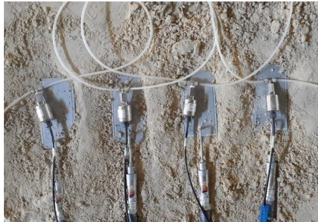
Fig. 2.6-1: Earth pressure cells and the settlement sensors.
