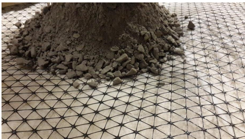
Figure 2.3-17: Installation of the GSY 3 and aggregates.
