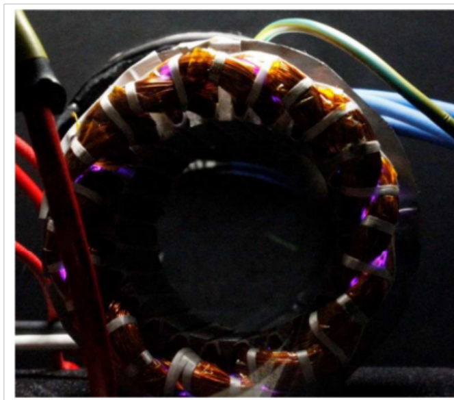
Figure I.32: Electrical discharges in stator windings [95] and [96].
