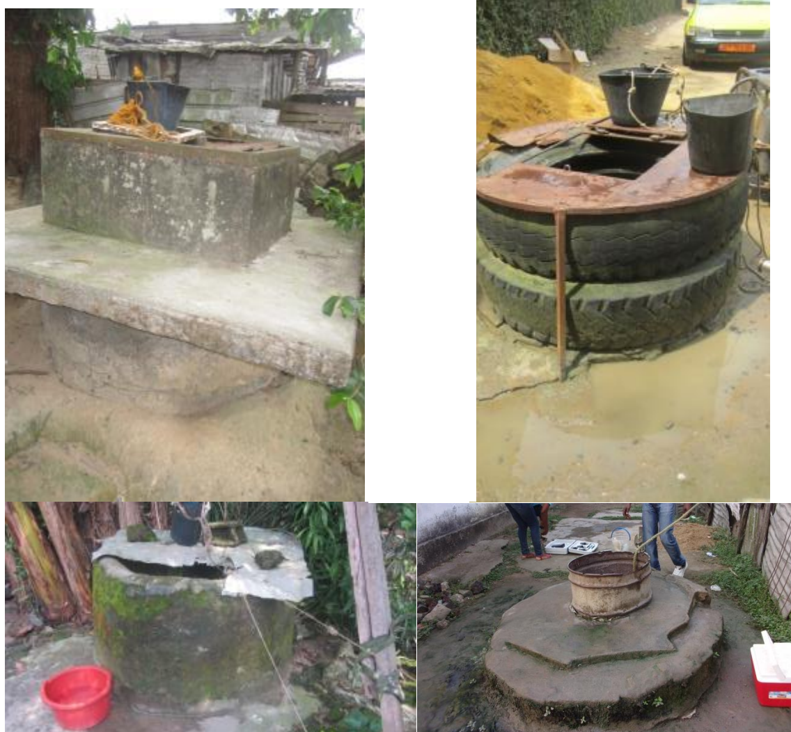
Figure 10: types of hand-dug wells in Douala.
