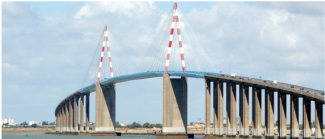
Figure 9.19: St. Nazaire Bridge (Janberg, 2020)
