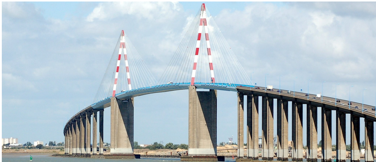
Figure 9.19: St. Nazaire Bridge (Janberg, 2020)
