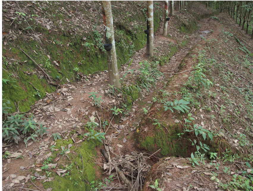
Figure 6.15: Formation of a gully in OR2 plantation. The rubber tree lines do not follow contour lines, creating concentrated flows and gullies.
