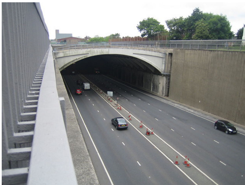
Fig. 1 Road tunnel coming upon a street canyon [9]
