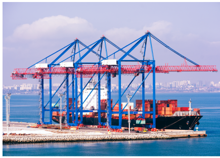
FIGURE 2.3 – Grue de quai
