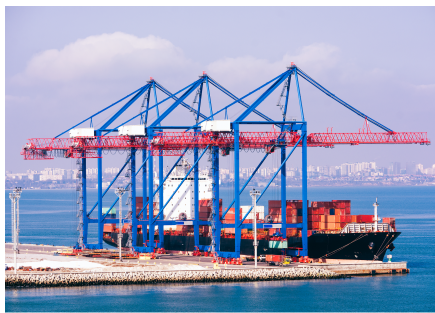
FIGURE 2.3 – Grue de quai
