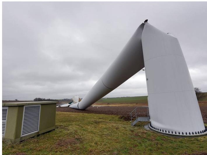
Figure 1.11: Collapsed wind turbine in Germany [The-Civil-Engineer, 2017].
