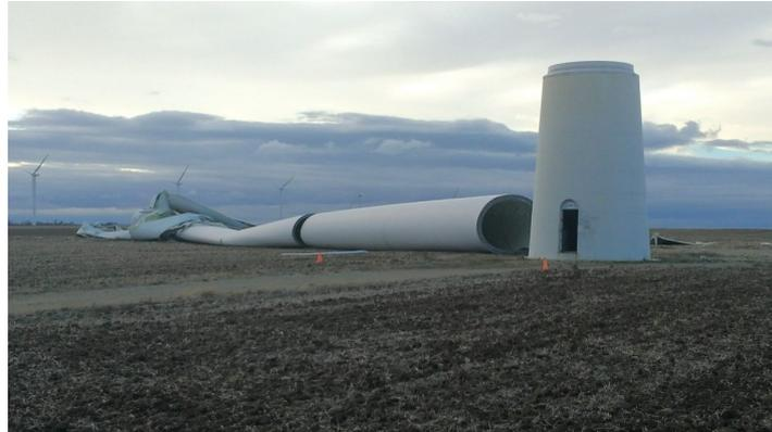
Figure 1.13: Collapsed wind turbine in Guineville, France [France-3, 2018].
