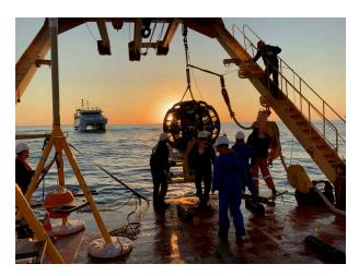
Figure 2.8: A picture of a DU deployment, where the detection unit is furled into the LOM.
