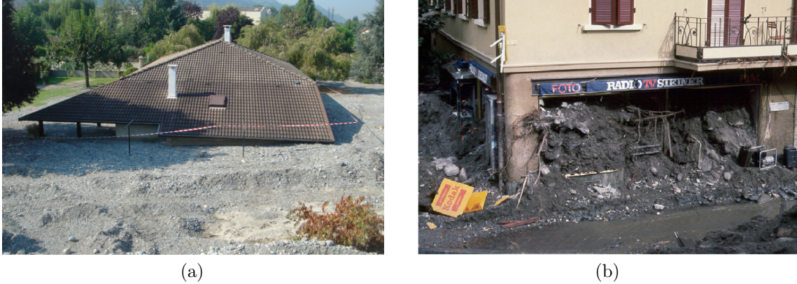
Figure 1.2: (a) Deposited sediment after the 2005 flood of the Domenon river in Domène (France). (b) Destroyed shop by the sediment transported by the Saltine river in Brigue (Switzerland). Credits for the pictures: P. Belleudy and R. Loat
