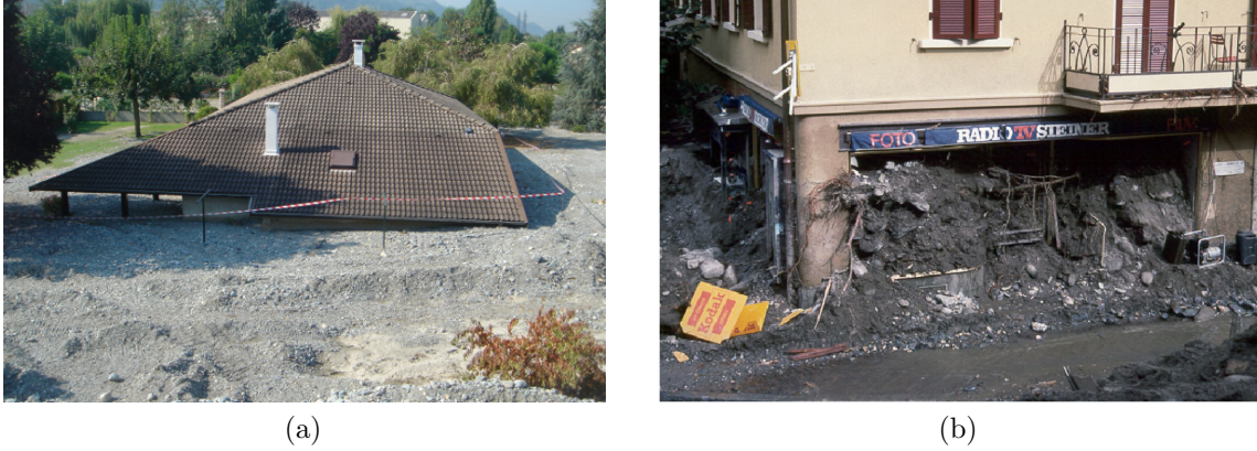
Figure 1.2: (a) Deposited sediment after the 2005 flood of the Domenon river in Domène (France). (b) Destroyed shop by the sediment transported by the Saltine river in Brigue (Switzerland). Credits for the pictures: P. Belleudy and R. Loat
