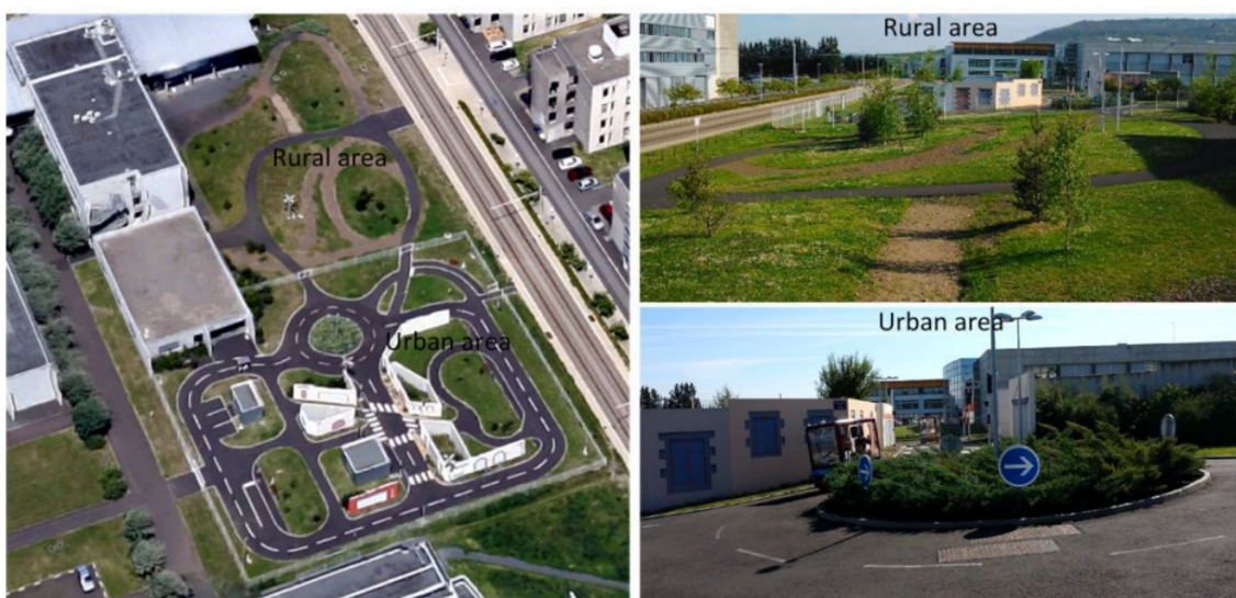
Figure 7.2: PAVIN experimental platform (Clermont-Ferrand, France)
