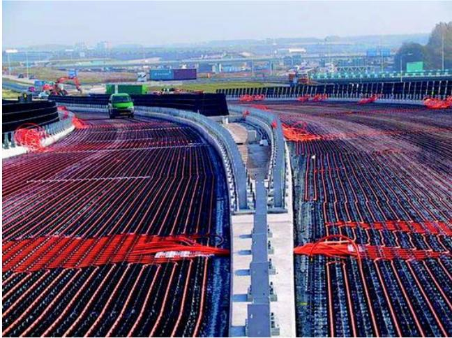
Figure 7. Layer of solar collectors along a road section [11].
