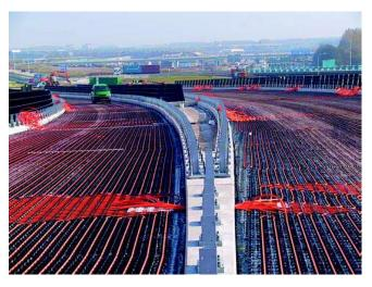
Figure 7. Layer of solar collectors along a road section [11].
